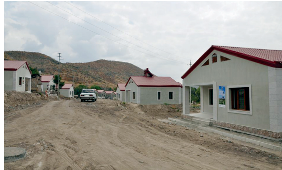
Newly established “Ariavan” settlement in the occupied Lachyn district, funded by Armenian diaspora from Lebanon through the “Artsakh Roots Investment Ltd.” | Photo from www.arirroots.com | 2014
