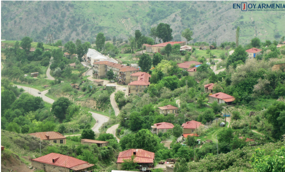
Newly constructed/renovated houses in the occupied town of Lachyn
