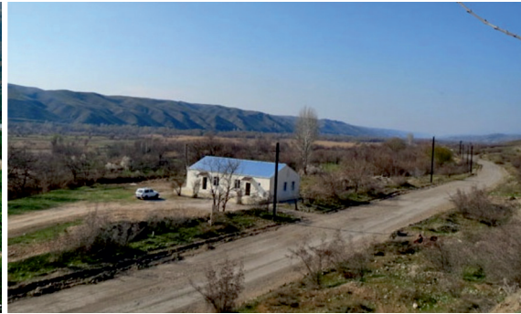
Two-apartment building for two Syrian Armenian families is built in Khanlyg village of the occupied Gubadly district by Tufenkian Foundation | Photo by Alvard Grigoryan | www.kavkaz-uzel.ru | 25 March 2014
