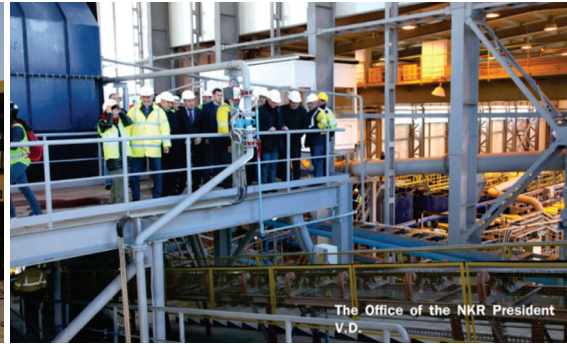
Commissioning of the ore processing plant at Demirli copper-molybdenum mine | Photo from www.artsakhpress.am | 26 December 2015
