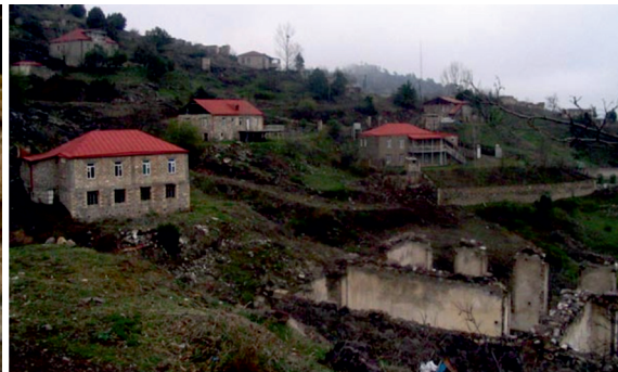
Newly constructed/rebuilt houses in the occupied town of Lachyn | Photo by Naira Hayrumyan | www.amenianow.com
