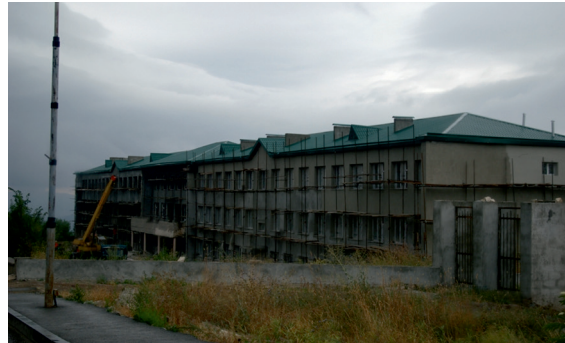
Construction/renovation of a residential building in the occupied town of Shusha
