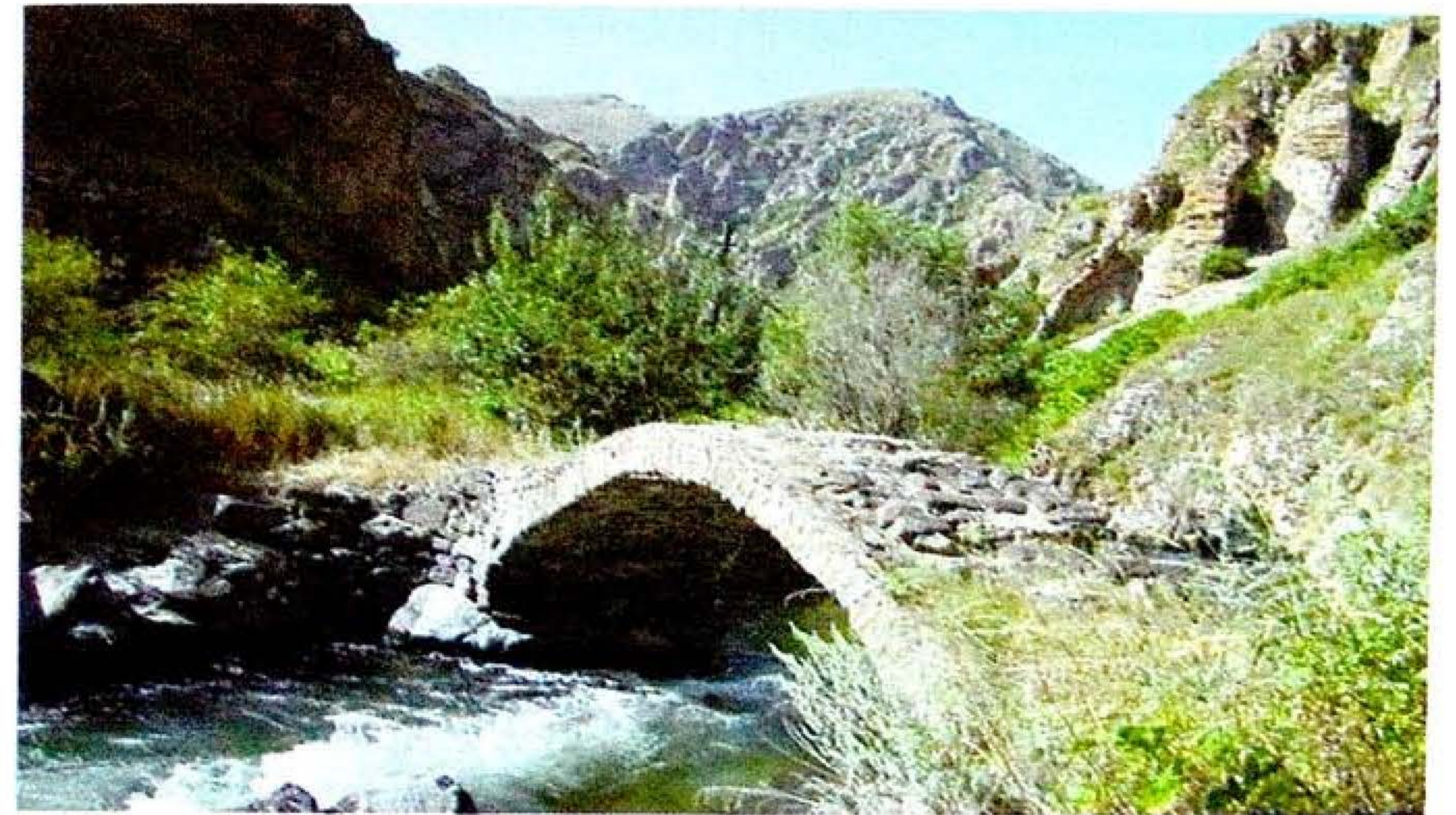
The bridge on the river Tartar in Kalbajar
